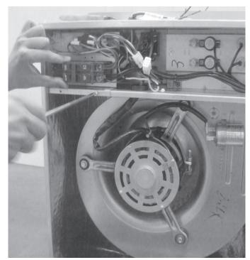
2. Remove the cover plate from the fan coil unit. Fix the heater kit instead of that and secure element plate with previous removed screws.
