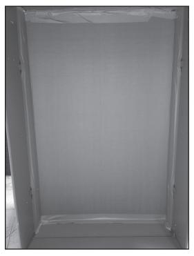
Please Note: This insert is intended to close the opening in the wall sleeve. It is not a permanent structure and will not prevent water/elements from entering the contractors work area.
