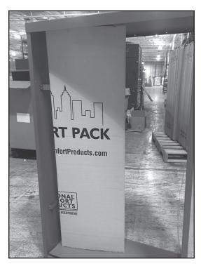
4. The insert should rest against the inside flanges of the wall sleeve
